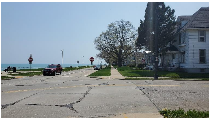
Looking South along Main St.
