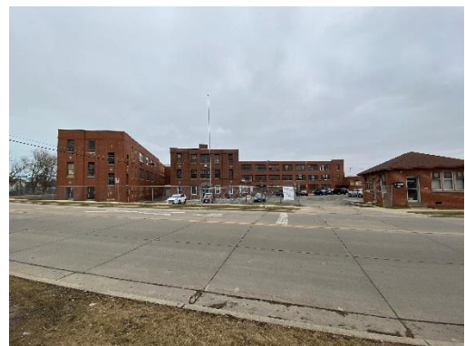
Looking south at east side of site
