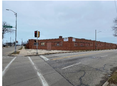
Looking south east at site
