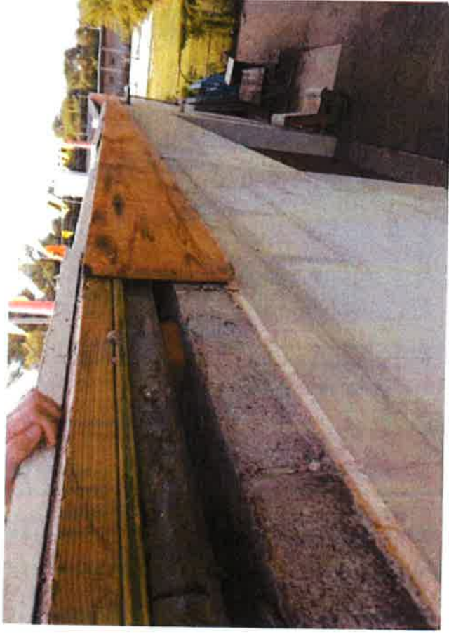
T&M for Gutter Edge Replacement
