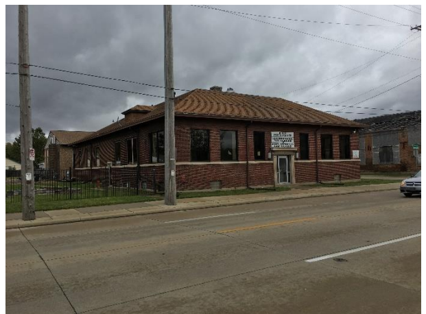
Looking west at original office building (1923) on property
