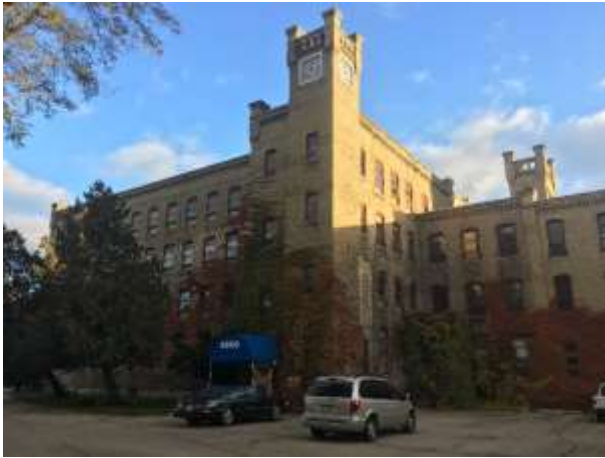
Looking north at 2200 Northwestern from front parking area
