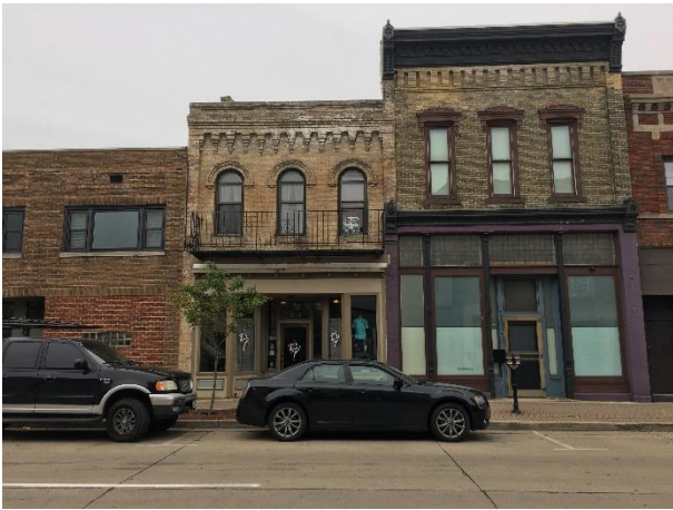
Looking south at subject property from 6 th Street
