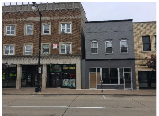
Looking north from subject property
