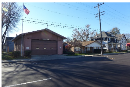
Front view of Fire Station 6
