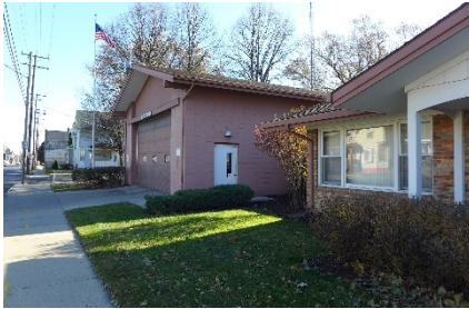
Fire Station 6 - Exterior
