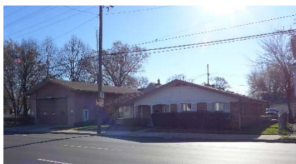
Front view of Fire Station 6
