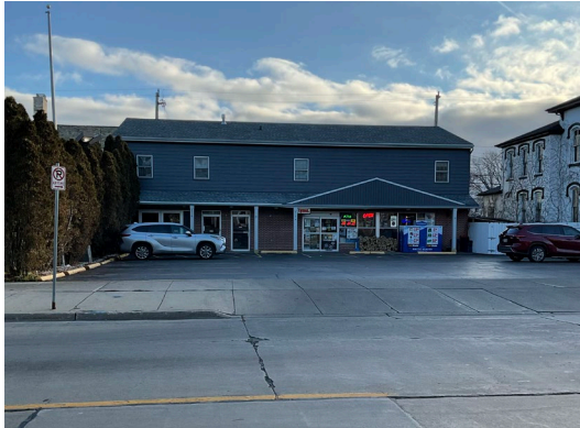
Looking east at subject property
