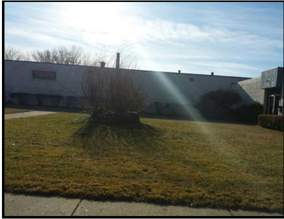
South view from site
