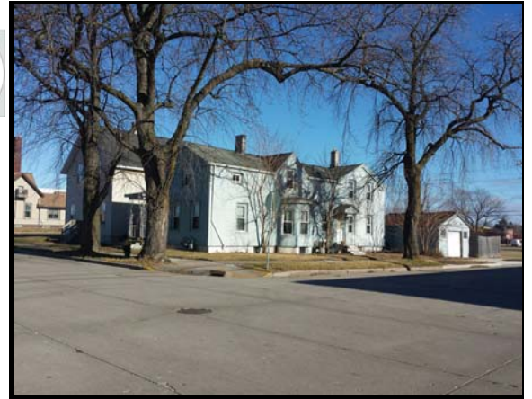
Northeast view from site
