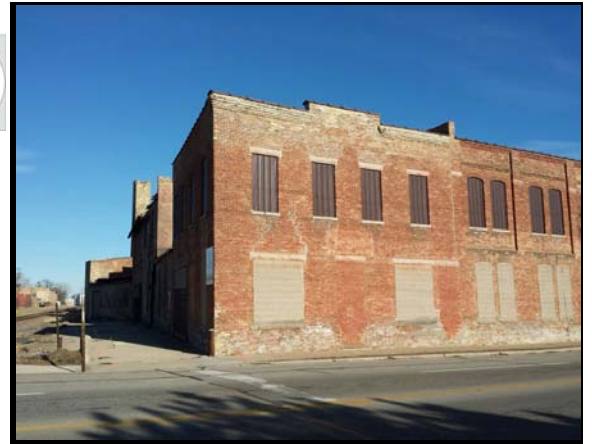
View of site from the southwest
