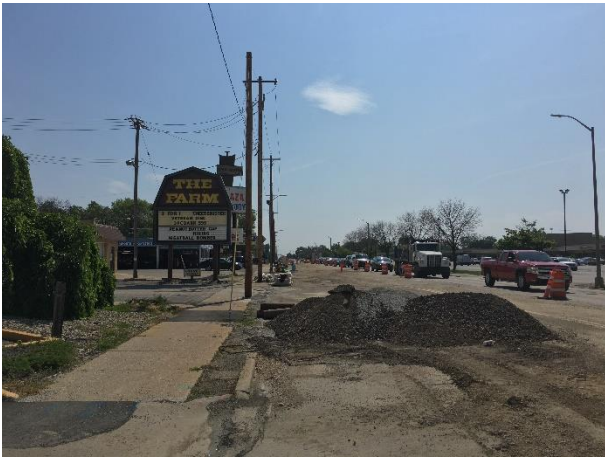
Looking east from the site down Durand Avenue
