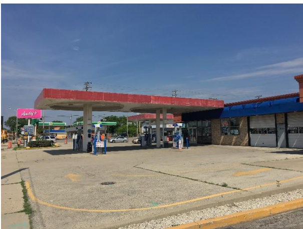
Looking at subject property from Durand Avenue
