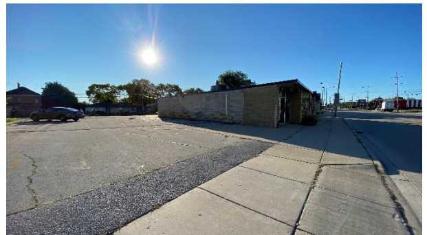
Looking southeast at building from Douglas Avenue
