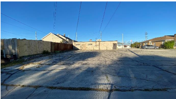
Looking west from rear of building
