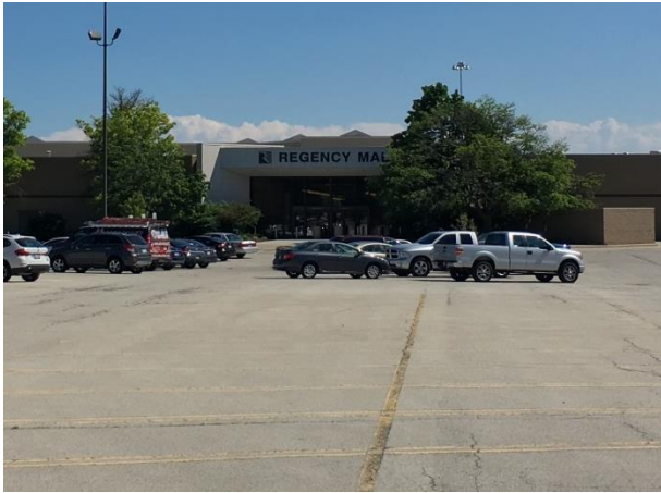
Example of mall entrance from edge of parking area
