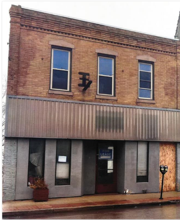
Current façade of 1346 Washington Avenue, picture provided by the applicant.
