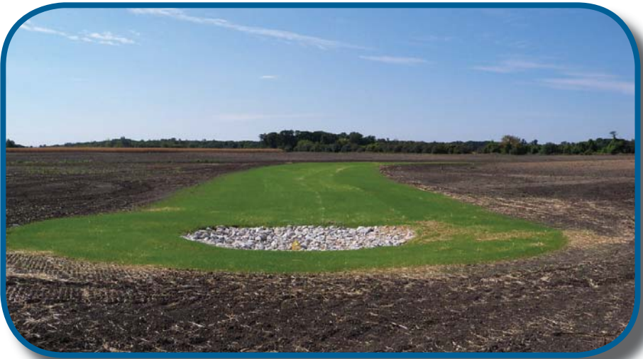
Pollution from agriculture can be reduced through best practices such as grass swales and inlets for collecting and filtering runoff.
