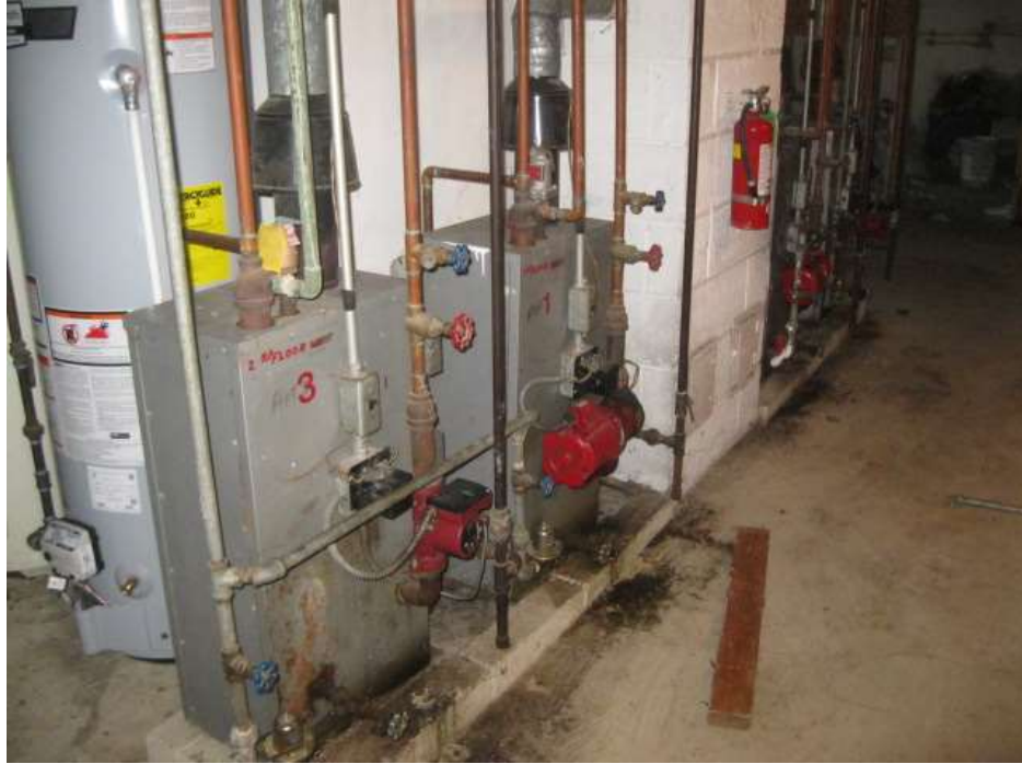
Interior View Boilers & Water Heater
