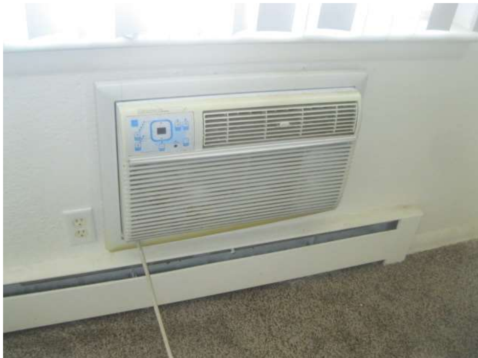
Interior View Sleeve Air Conditioning
