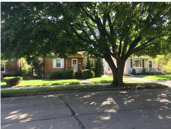
Looking at the front yard of the subject property
