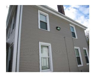
1224 Grand needed removal and replacement of deck boards on the front porch and stairs. Siding also needed to be removed and replaced between the windows on the north side of the home, which was riddled with holes from a woodpecker. The home was completely pressure washed, and replacement stair parts and siding were painted to match the home.
