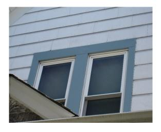
This aluminum sided home was a late addition to the project. After receiving a citation from the City of Racine for failing siding and trim, this homeowner contacted RRP for help. The home required that the fascia on the front gable be removed and replaced. Also, the metal on the upper front window was removed and replaced. The aluminum was painted to match the existing color of the home.
