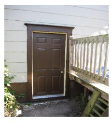
1200 Grand required work on the foundation at the front and sides of the home along with work on the front porch. An entire house painting with trim was done and the contractor replaced the rotted areas at the porch and installed new lattice on the front of the home. The side deck had loose boards that were replaced and secured and a new basement door, visible from the street, was installed.
