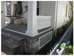
1232 Grand is a charming small home, needing several porch repairs to include a new bull nose around porch, and crown molding on the front porch. Replacement of bad deck boards and soffit. The lattice was also removed and replaced. The contractor installed new joist hangers on all joists to support the weight of the deck. Repairs under the porch were also made to support the beam with a 4×4 post.
