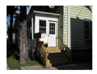
and replacement of 6 existing porch windows which were cracked, broken and inoperable. Removal and installation of new treads and risers on steps and new handrails on both sides of the stairs. A new front door was installed. The door and windows were supplied by the homeowner in order to make this project fit the program budget.
