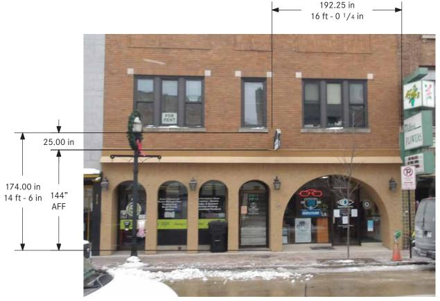
EXISTING SIGN (EYE): 46.5 (L) x 16.75" (H) x 3.5" (D) ▲ EXISTING EXISTING SIGN (TAGLINE): 46.5 (L) x 11.5" (H) x 3.5" (D) EXISTING MOUNTING BRACKET: 18" OAH; 10" SPACE BETWEEN TOP AND BOTTOM BRACKET
