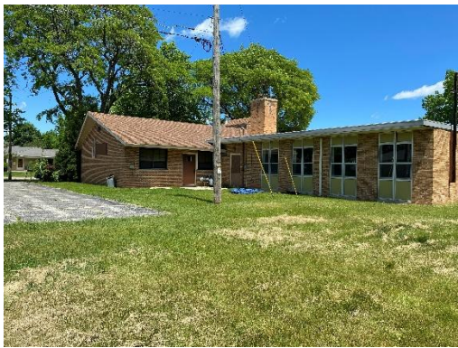
Looking Northeast at site
