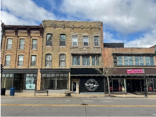
Looking West at front of building
