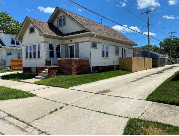
Looking Southeast at existing house
