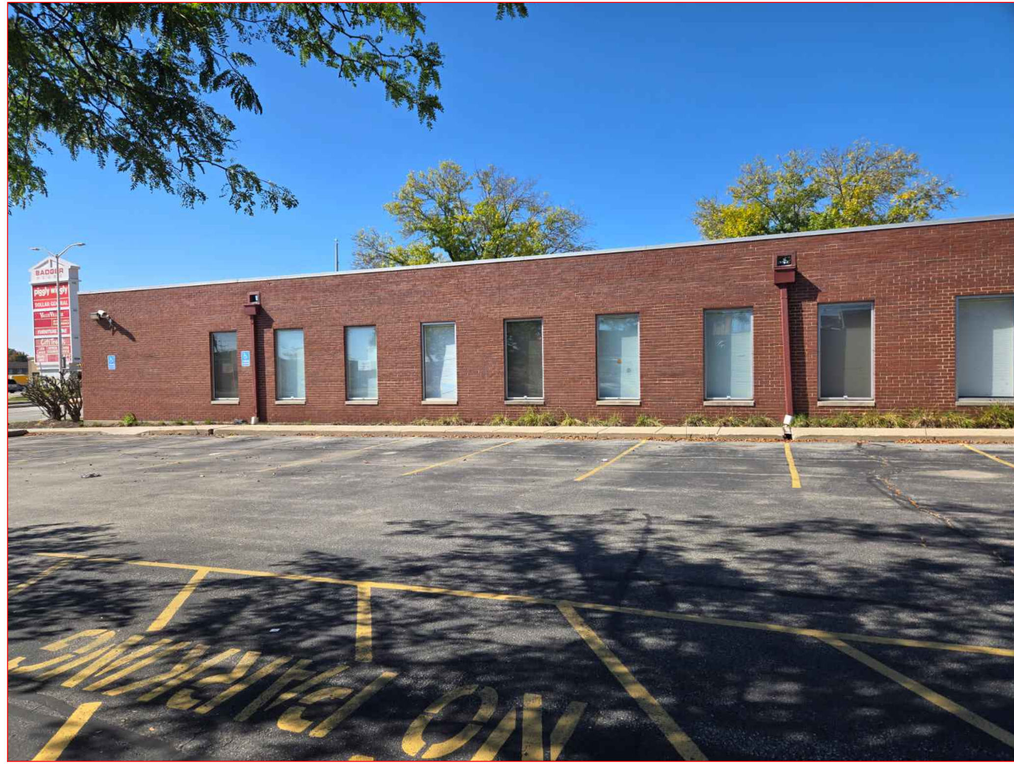
EXISTING BLDG EAST
