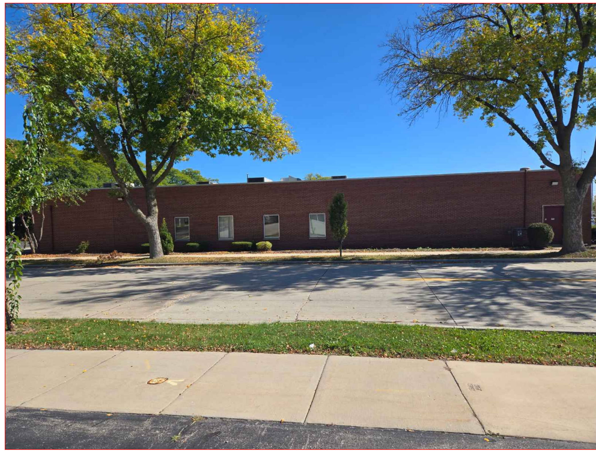
EXISTING BLDG WEST
