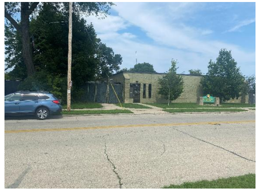
Looking North at existing administrative building
