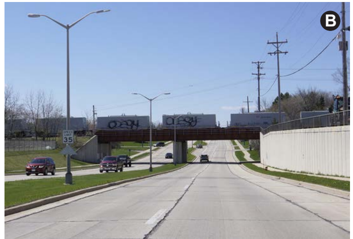
Above, photograph, from April 2024, of the the two-span bridge over College Avenue shows freight cars with cargo stored on a siding track. The highway grade is depressed to pass under the track. Below, September 2025 photograph of stone arch faced bridge over Oak Creek Parkway.
