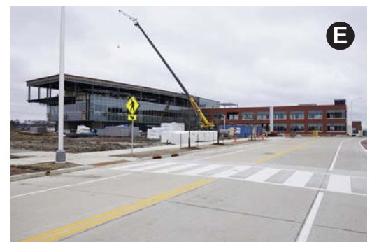
Innovation center under construction at KIN
