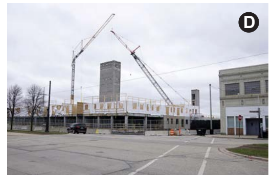
Apartments under construction, major project in downtown
