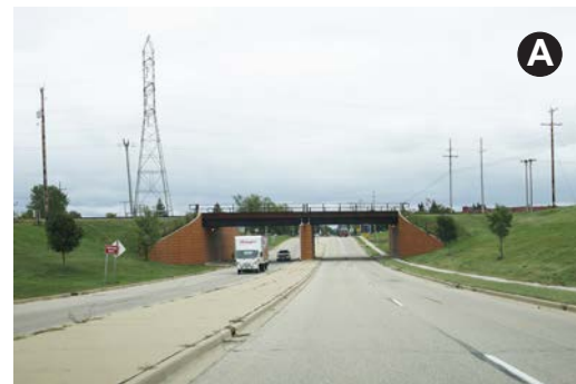
MARK Rail bridge over Four Mile Road
