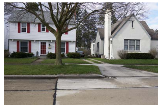
Single-unit houses in north Racine near the lake
