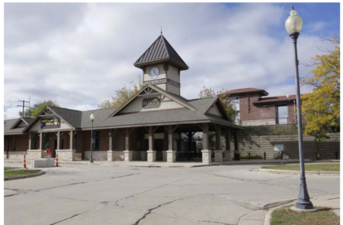
The front facade of the Kenosha Metra Station showing its 2010 renovation.
