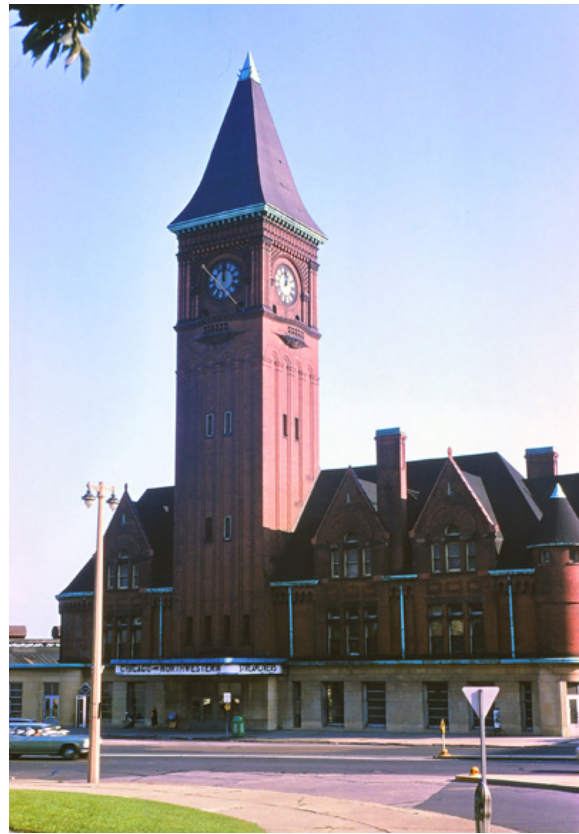
C&NW's Lakefront Depot photographed in 1965, after service was abandoned and the property sold to Milwaukee County. Photo credit: Ray Szopieray (courtesy of Karl Bandow and OnMilwaukee.com)
