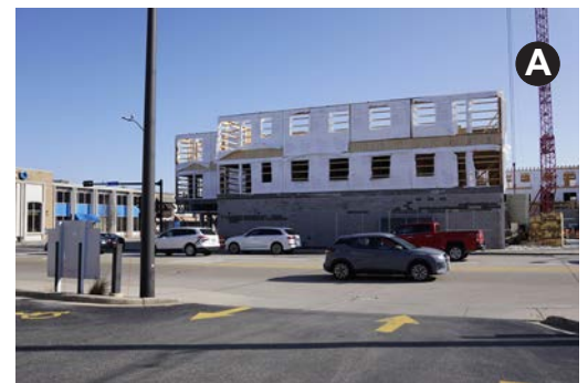
New construction, corner of Layton Avenue and Packard Avenue
