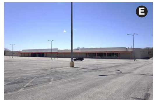
Former Kmart site, located immediately east of track
