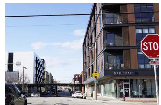
New loft residential and CPKC elevated track over 2nd Street at Florida Street
