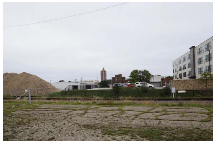
Photo from Junction Avenue shows the proximity of MARK Rail track to SC Johnson’s office tower a quarter mile to the east.
