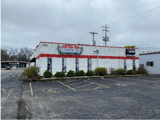
Looking East at subject property
