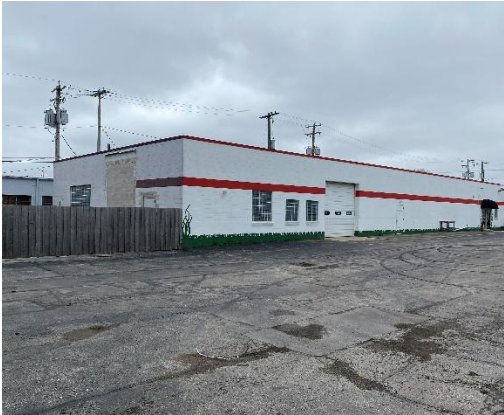
Looking Southwest at subject property
