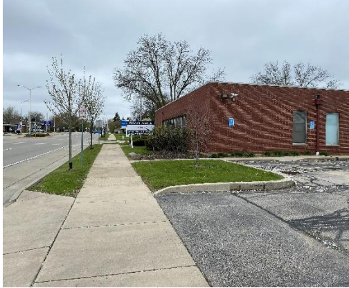
Looking West at front of subject property
